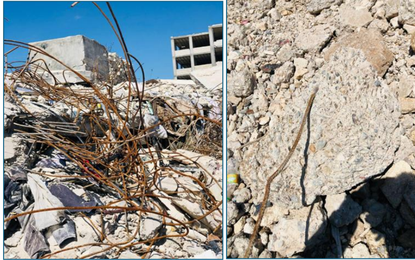
Figure 4. Adhesion weakness in reinforce bars
