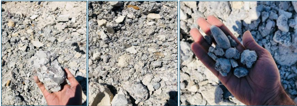
Figure 3. Incorrect granulometry usage observed in concrete and the use of river-sea aggregate
