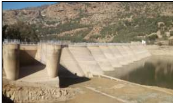
Figure 1 : BENI-BAHDEL multi-arch dam.
