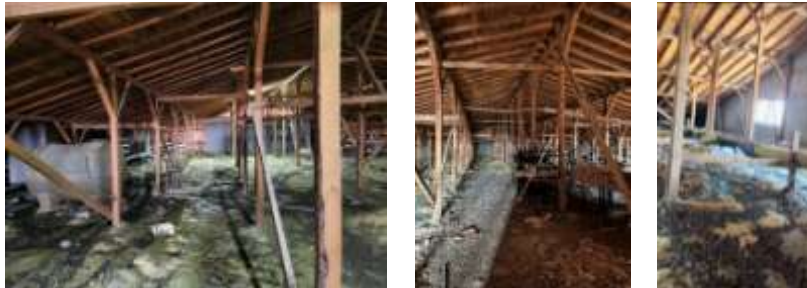
Figure 3. Selçuk University Faculty of Architecture and Design Rooftop visuals (Sungur, 2023)
