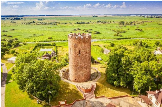
Kamenets Tower today
