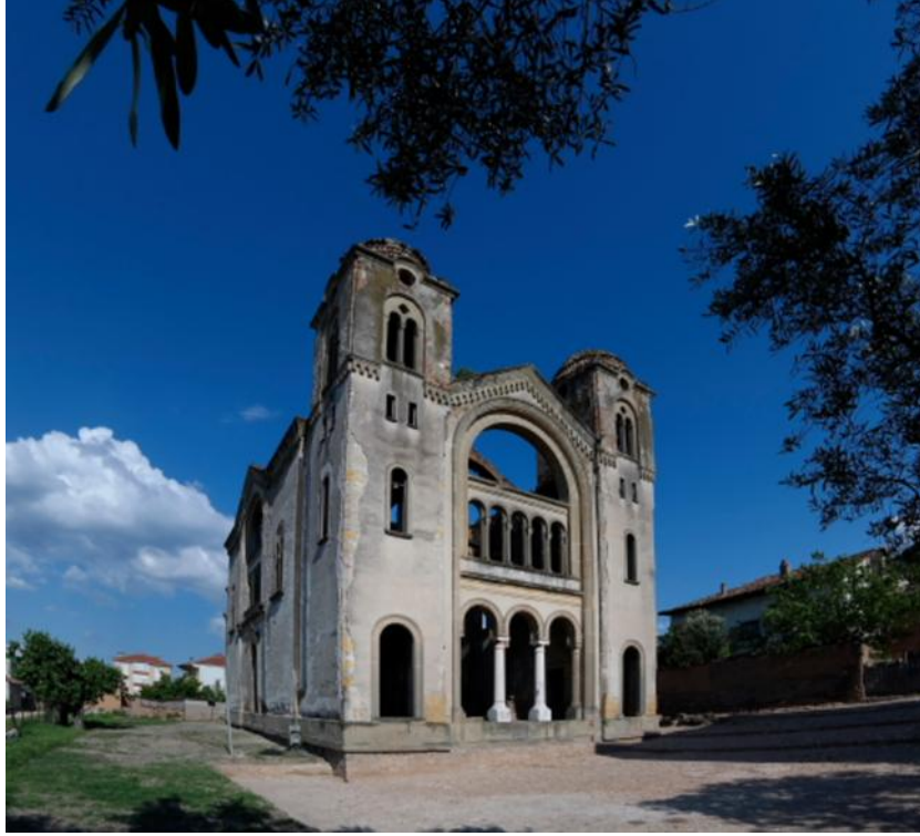
Figure 2. View of Hagia Yorgi Church ( https://www.osmaneli.bel.tr/hagios-georgios-kilisesi )
