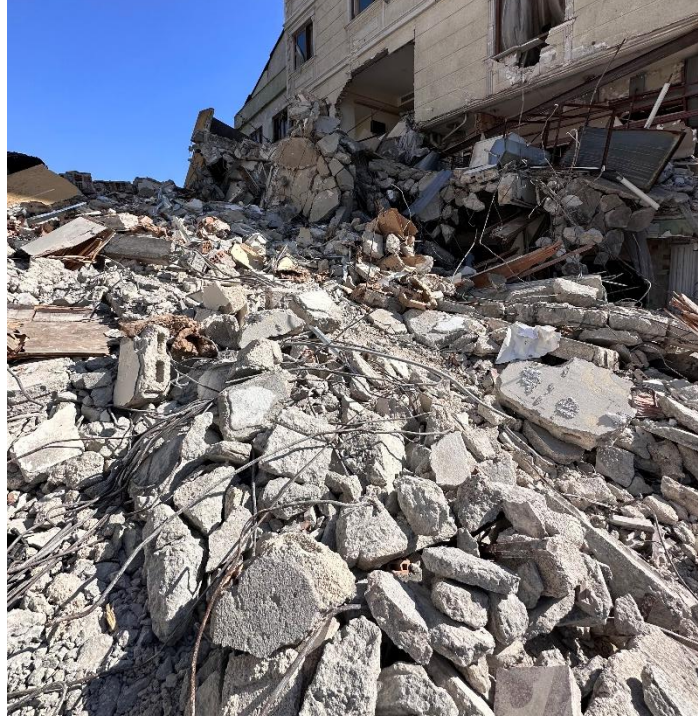
Figure 3. Concrete waste post-demolition (Kamanli et al., 2023)
