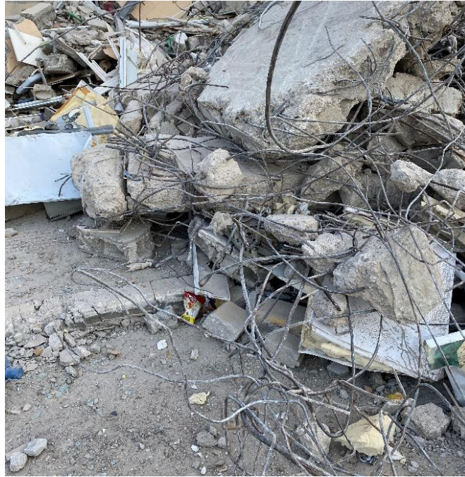
Figure 4. Metallic waste from demolitions (Kamanli et al., 2023)
