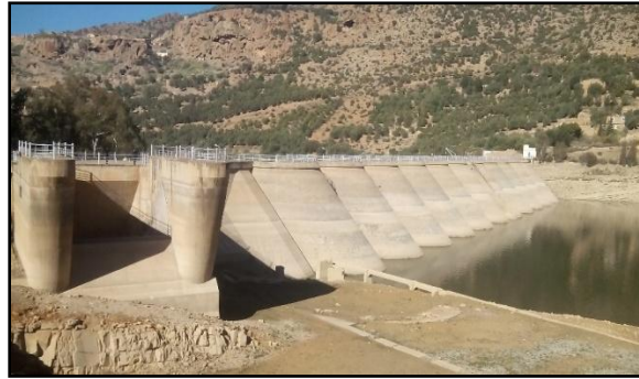
Figure 1 : BENI-BAHDEL multi-arch dam.
