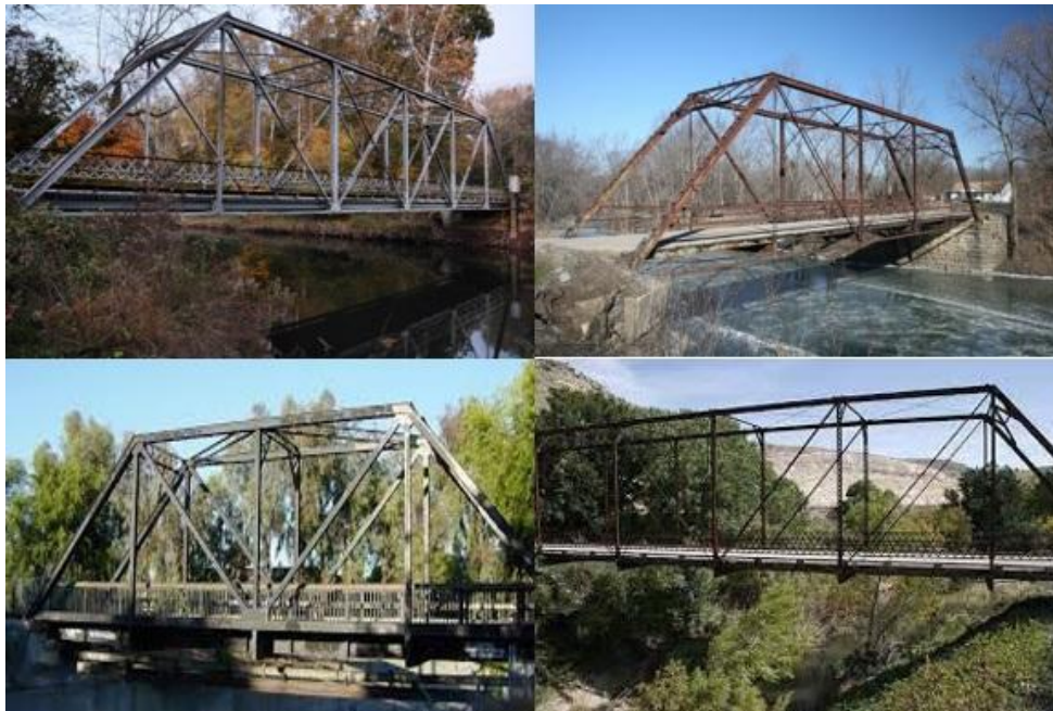
Fig. 1 Examples of truss type steel bridges
