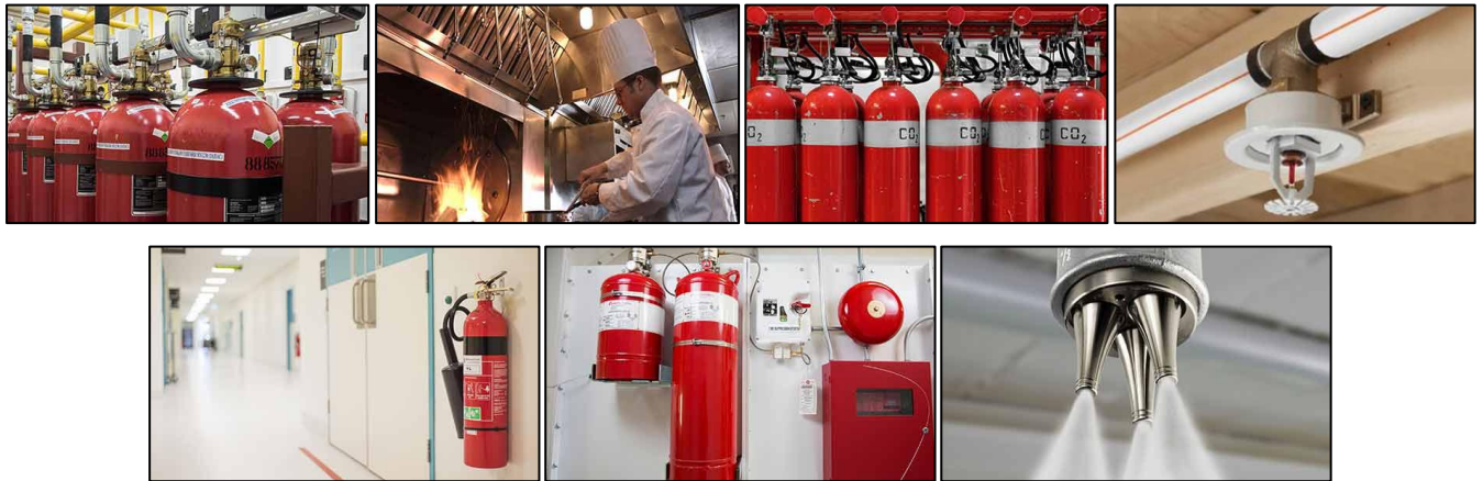
Figure 1. Fire suppression systems (Fm 200 Extinguishing Systems Hood Extinguishing System, Carbon Dioxide Extinguishing System, Sprinkler Extinguishing System, Foam Extinguishing System, Internal Extinguishing Systems, Water Mist Extinguishing Systems)
