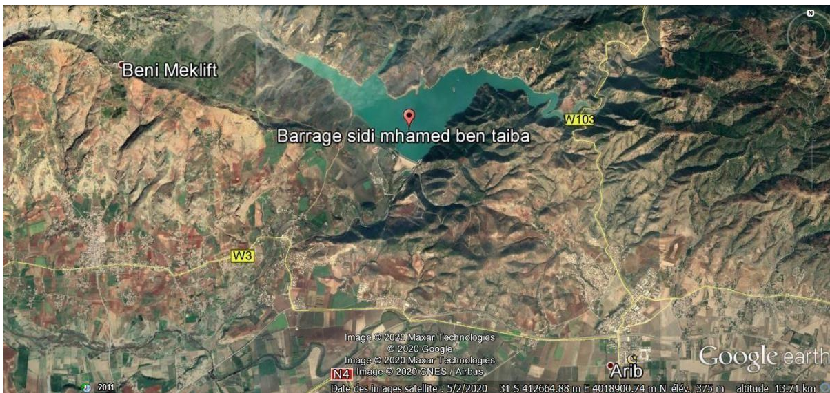
Figure : View of the Sidi M'Hamed Ben Taïba dam (Google earth,2020)
