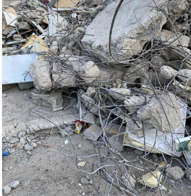
Figure 4. Metallic waste from demolitions (Kamanli et al., 2023)
