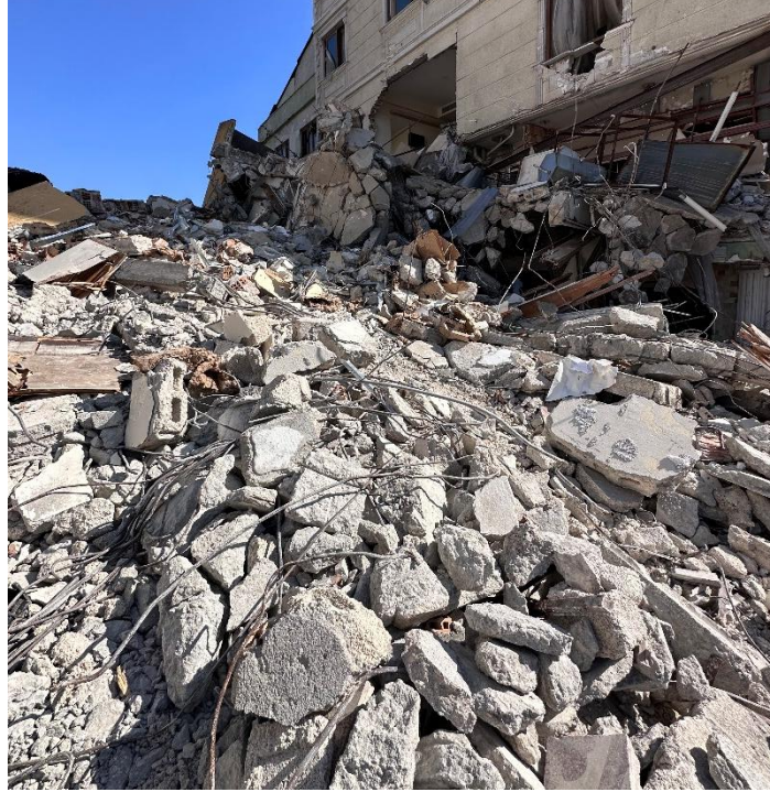
Figure 3. Concrete waste post-demolition (Kamanli et al., 2023)
